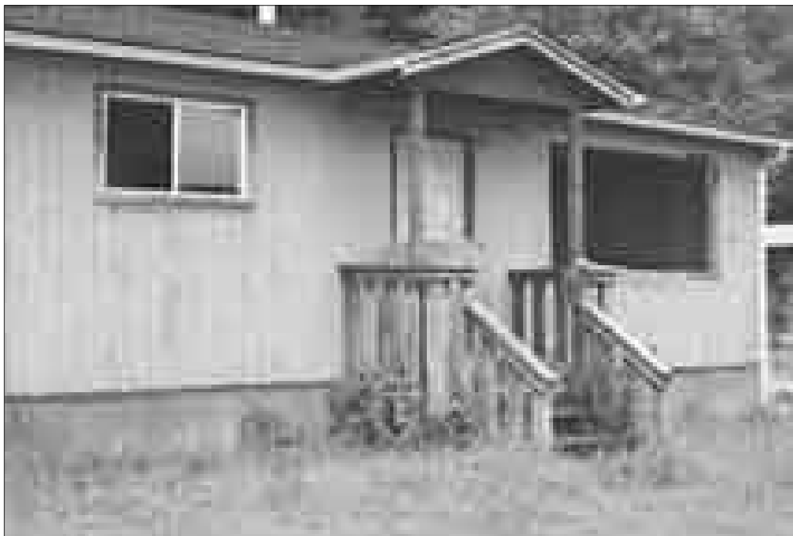
Indian Reserve house with missing windows on Guilford Island, BC.
