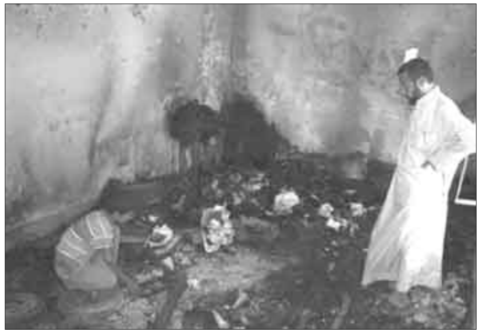
A house damaged during US bombing raid in Fallujah, September 2004.
